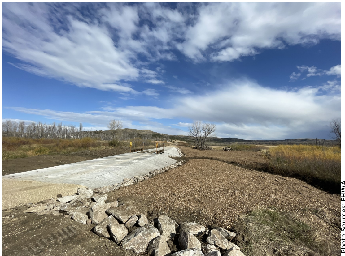
Completed Bridge Installation and Armored Concrete Pavement Crossing at Rock Creek.
