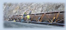
A 240 TON Crane was used to place the side rails of the bridge and then it was bolted in place.
