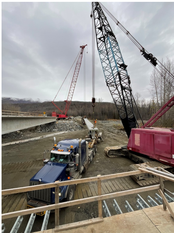
Upper Right: Cranes lifting girder Lower Left: Lifting a girder from the delivery truck Lower right: Setting girder in place
