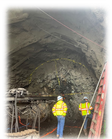
Left & Right: East Portal line drilling
