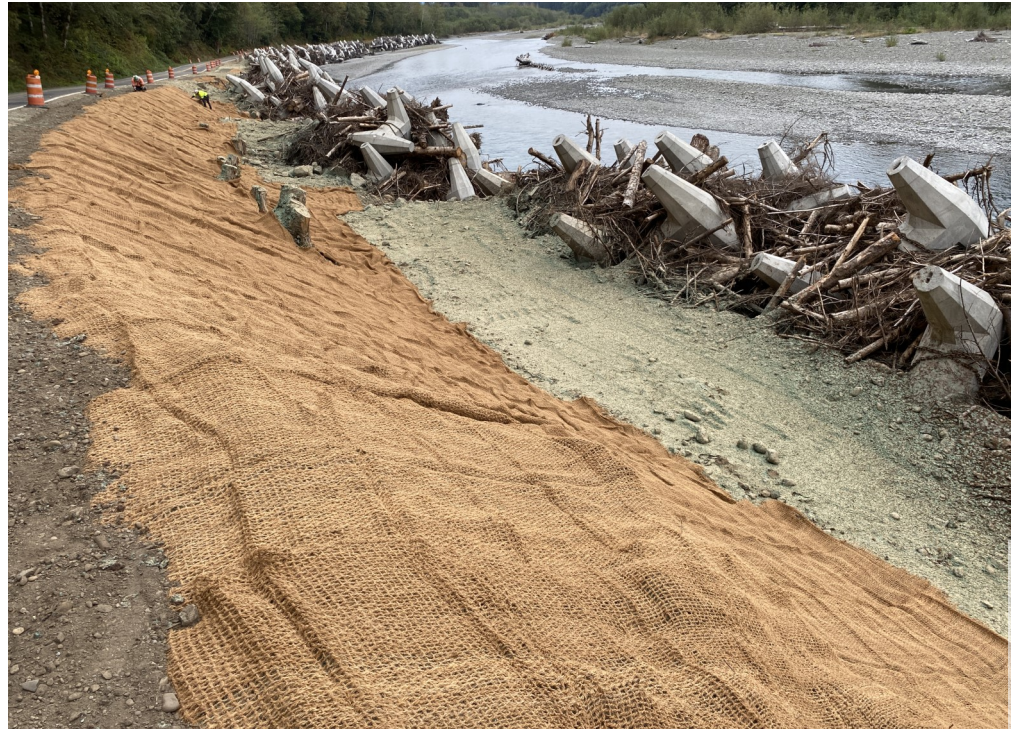
Rolled Erosion Control Product installed on the slopes at the MP 4 ELJs
