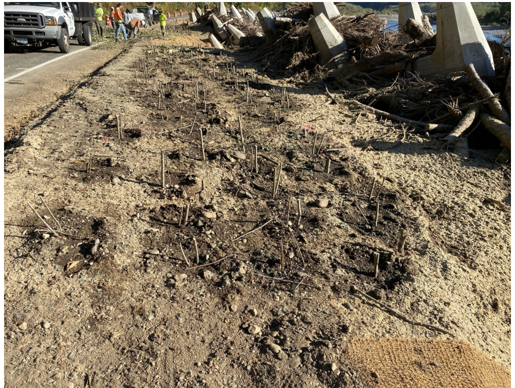
Willow and Cottonwood pole plantings installed at the MP 4 ELJs
