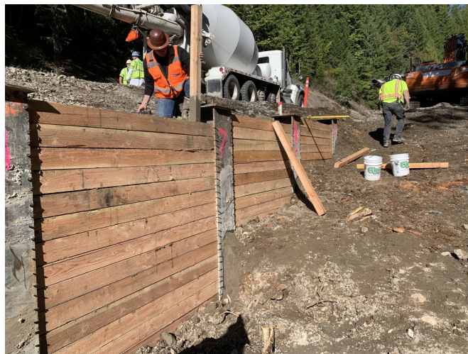
Photo left: Shows Timber lagging and lean concrete backfill Sta 75+48. All images Source: FHWA
