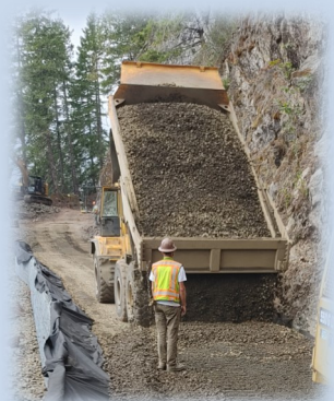
Preparing subgrade & adding road aggregate
