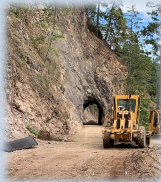
Preparing subgrade & adding road aggregate
