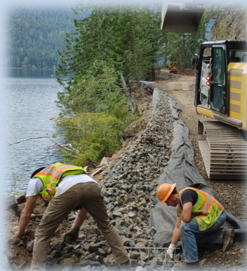
Adding a wall on the west side and removing root wads
