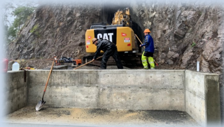
Backfilling the abutment
