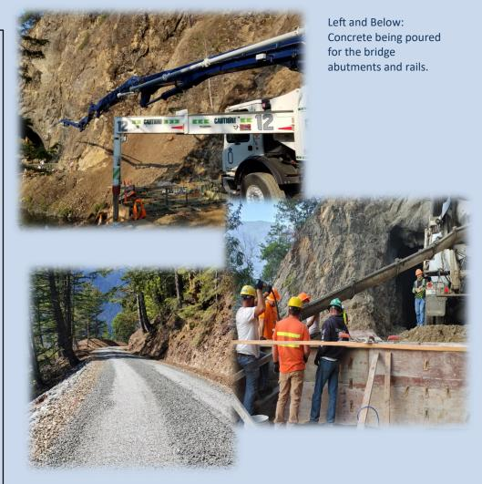
Above: Aggregate being placed in preparation for the pavement surface in between the two tunnels.
