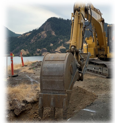
West bench outlook retaining wall excavation
