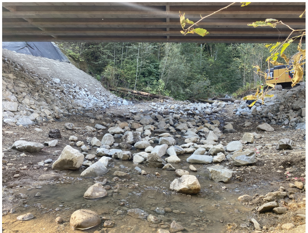
Reconstructed streambed under Tower Creek Bridge
