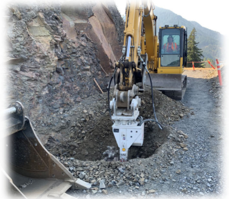
West bench culvert excavation
