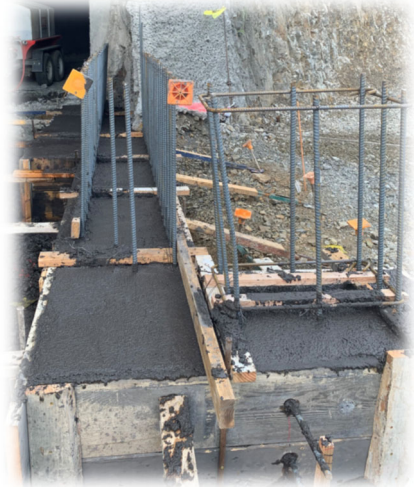
East portal wing wall foundation concrete pouring
