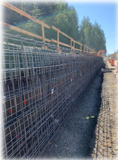
Rebar at Dome Rock MSE Wall
