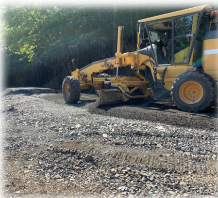
Blading grading material into place
