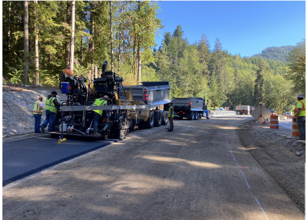
Paving the asphalt at Tower Creek MP 7.8
