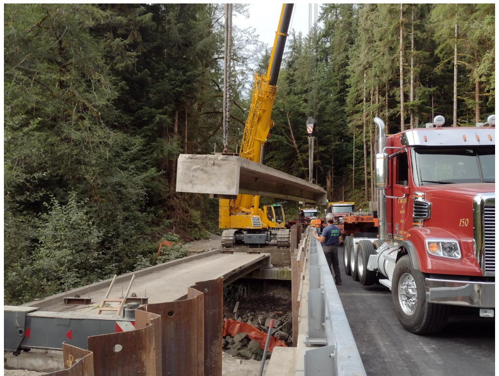
Removing the remaining girders of the old Tower Creek bridge
