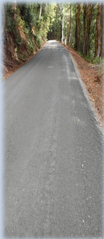
Placement of road aggregate base before asphalt
