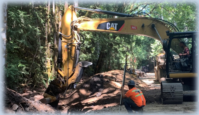
New culverts being installed.
