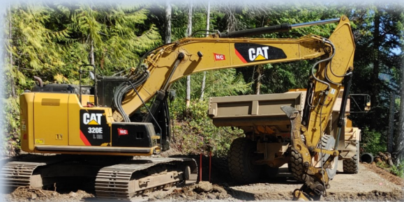
Above: Excavating for Culvert to be installed
