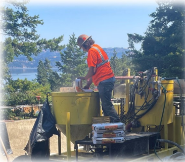
Above and Right: Mixing and testing grout for anchor bolts
