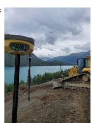
As DCC excavates, a bench of material is left to later serve as a platform for equipment to sit when installing the underdrains on the slope.
