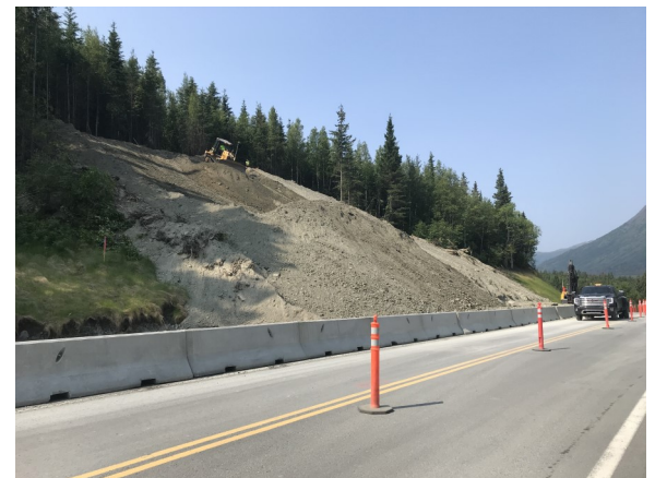
Dozer cutting slope at Sta 315+00.
