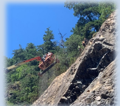
Left and Right: Mesh continues to be installed.
