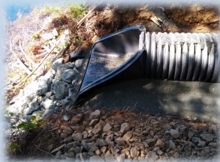
Installation of new Culvert
