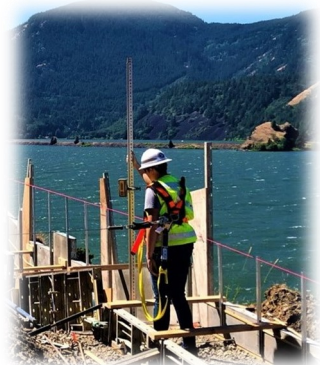
Wall footing grade check
