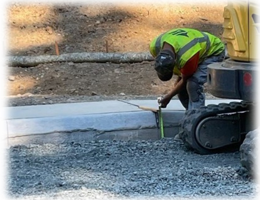
Right: Measuring curb for grading
