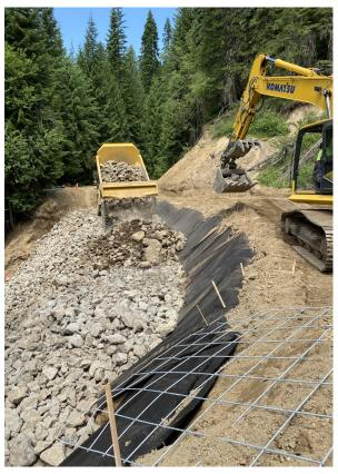
FSR 426 MP 0.5 Special Rock Embankment wall nearing completion
