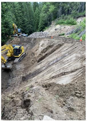
FSR 426 MP 0.5 ongoing excavation and stockpiling of rock for Special Rock Embankment wall
