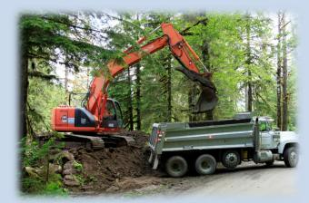
The Contractor has mobilized the majority of their equipment and began removing the debris flow stockpiles from previous storm events. Located at Forest Service Road 20 (Mountain Loop Highway) Mile Post 35.4.
