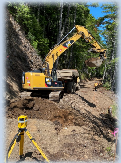
Right: Excavating for walls
