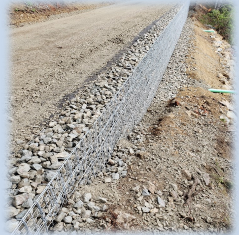
Construction and completion of 4th MSE Wall
