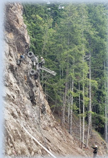
Wagon drill on US40 slope on the Eastside of the tunnel
