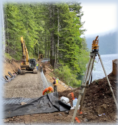
Construction and completion of 4th MSE Wall
