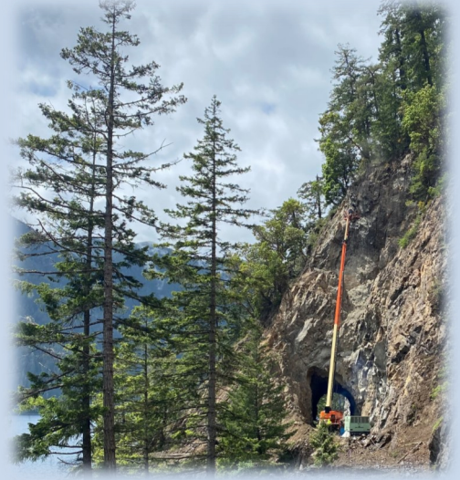
Wagon drill on US40 slope on the Eastside of the tunnel
