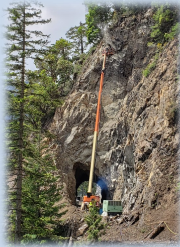
Drilling continues on the Eastside of the Daley Rankin tunnel. Crew is constructing the 3rd and 4th walls.
