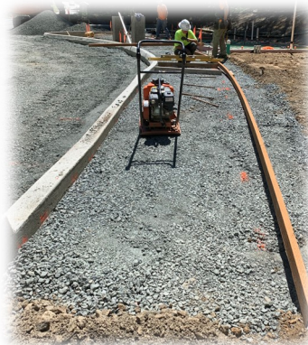
Left middle: Sidewalk prepped for concrete
