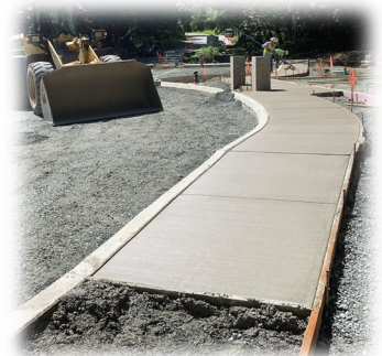
Right middle: Concrete poured
