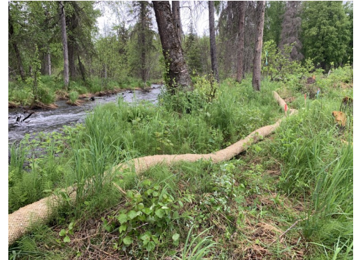
Above: Straw Wattle Installation
