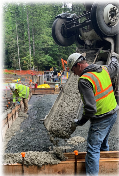
Right: Pour- ing concrete for Variable Message Sign foundation
