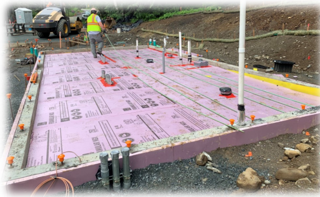
Left: Placing rebar for floor slab.
