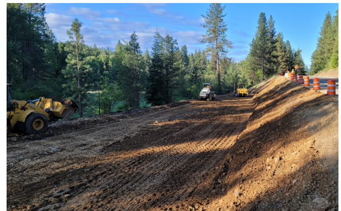
Embankment construction
