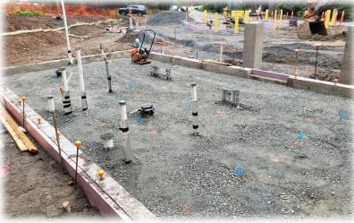
Left: Yellow bollards, two concrete columns for canopy in front of building, plumbing and electrical installed and filled with gravel.
