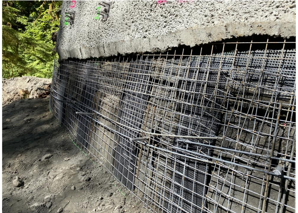
Rebar and drainage system installed around the nails prior to shotcrete
