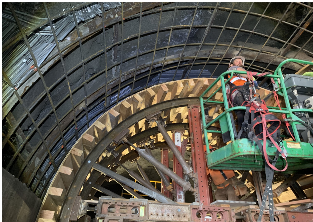
West Portal Concrete Structure Support Assembling
