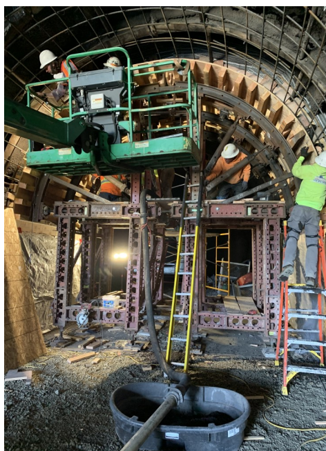
Concrete Pouring at West Portal Arch
