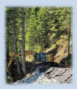
Clearing and excavating debris from the trail to complete the 3rd and 4th walls. Placed riprap on the slope and drilling continues inside the tunnel and on the rock face to install rock bolts.
