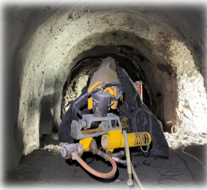
Shotcrete robot set up
