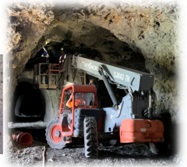
Adit #3—replacing spider plate #9 rock bolt
