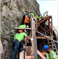
**Below Left**: Reinforced Steel Forming at East Portal Parapet **Below Right**: Prefabricated Pilelaster Cap Installation at West Bench
