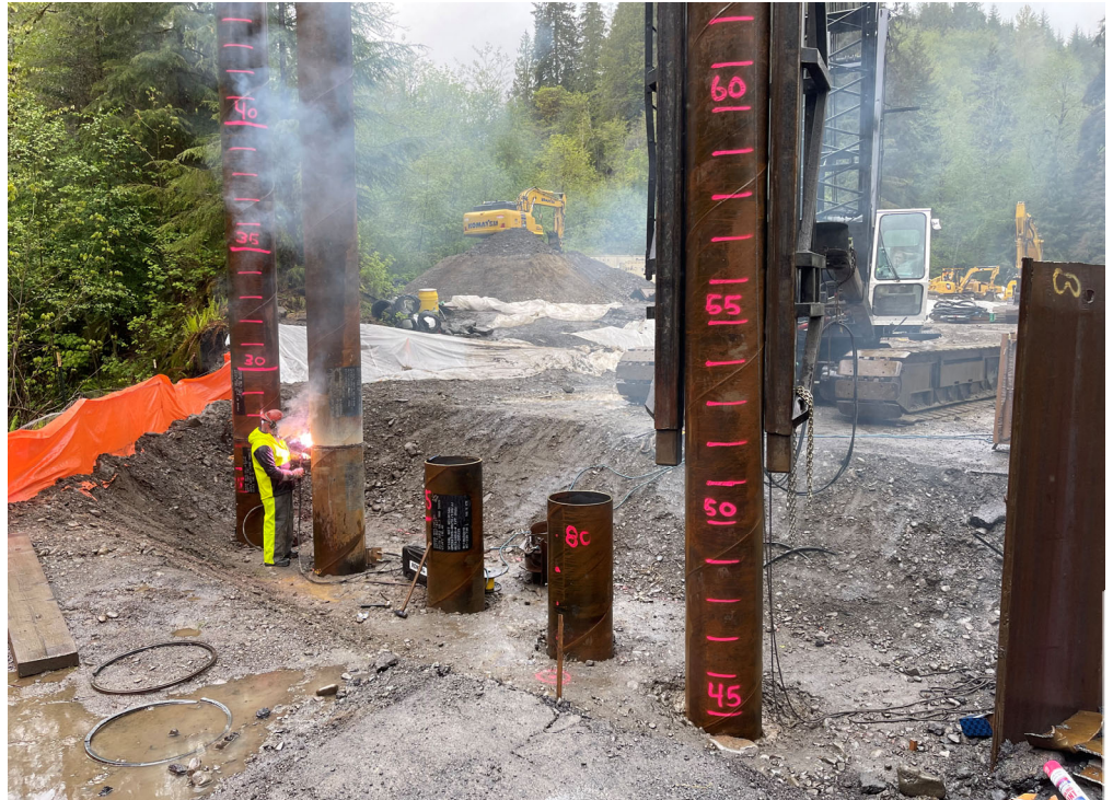
ICI subcontractor installing 24" steel pile foundation
