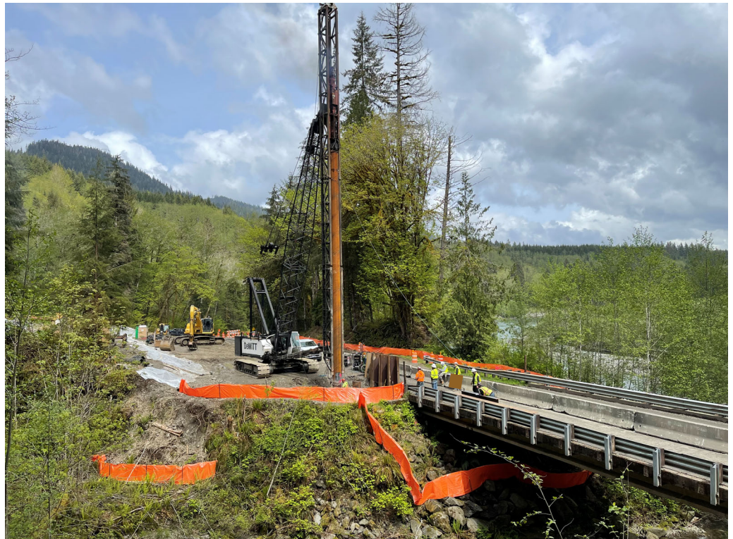
ICI subcontractor installing 24" steel pile foundation
