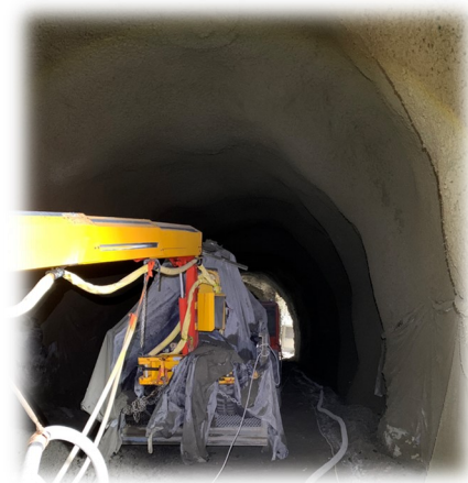
Shotcrete spraying at Adit #5 to Adit #4
