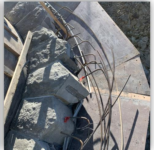
**Below Left:** Structure Arch Concrete Rebar and Form Work in East Portal
