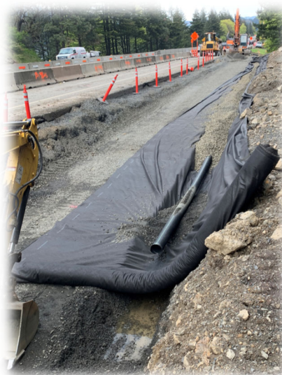
Back drain installation at Ridge Cut MSE wall
