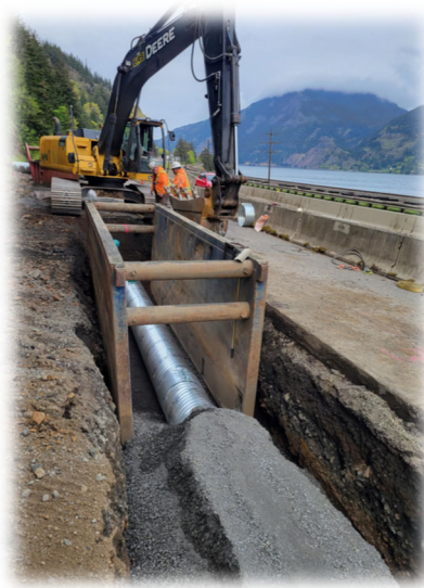
Back drain installation at Ridge Cut MSE wall
