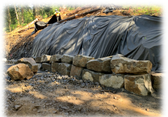
Placed boulders for rockery wall
