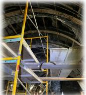
Below Left: Stone veneer grouting in East portal arch, Below Center: Stone masonry South Side, Right: East portal arch stone masonry North side
