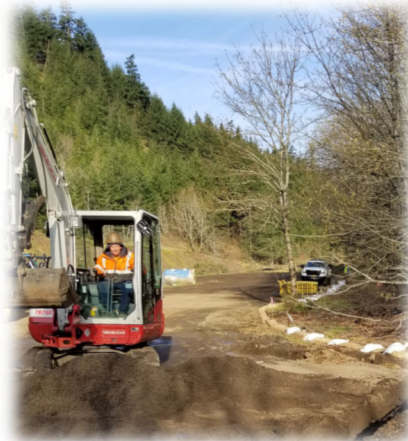
Left: Placing temporary Culvert for drainage
