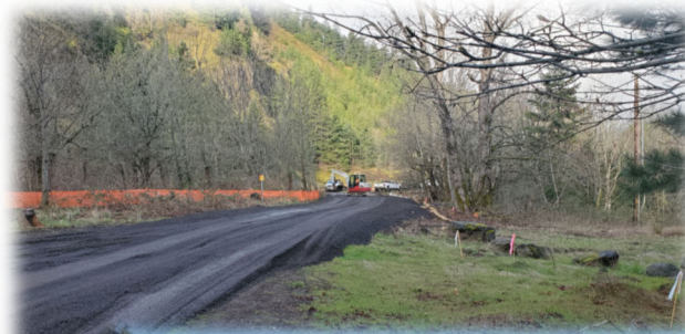
Left: Installing aggregate at the Construction Entrance
