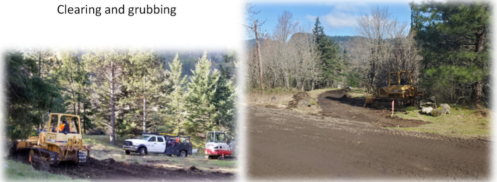
Left: Installing aggregate at the Construction Entrance
