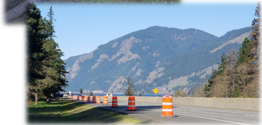
Below: Installing Traffic Control for access to site
