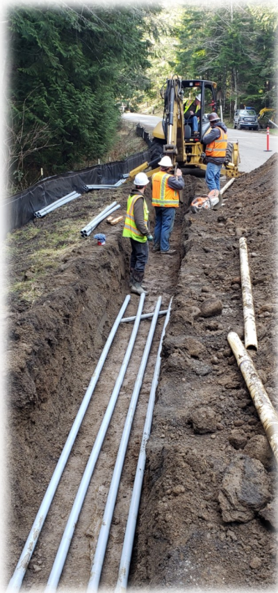
Duct installation for Fiber Optic
