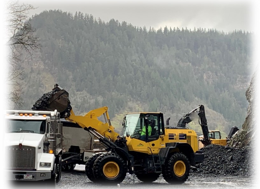
West tunnel mucking from Mitchell Point parking lot
