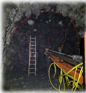
West tunnel drilling by two boom jumbo drill
