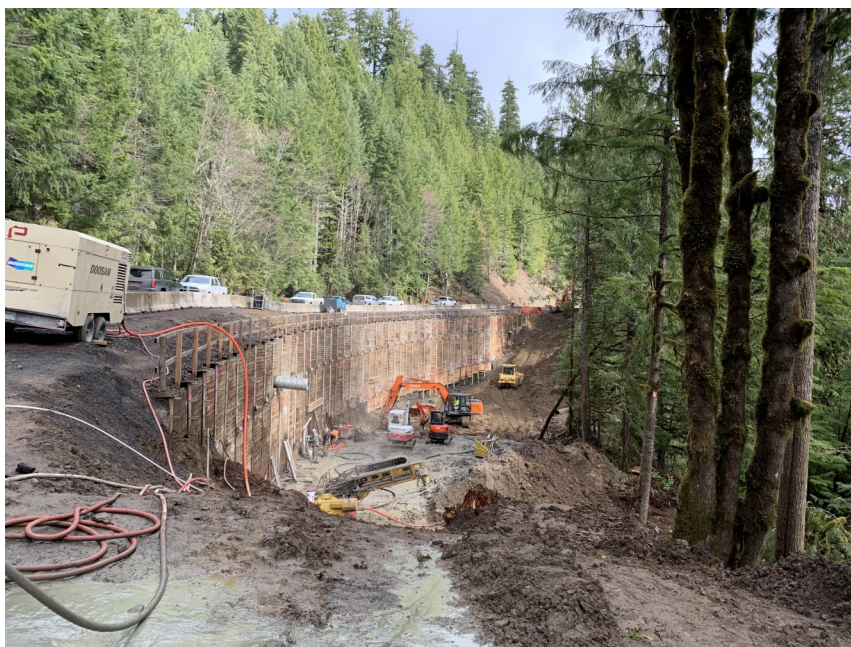
Photo left: Shows Finished drilling ground anchors and excavation. at MP 56. All images Source: FHWA
