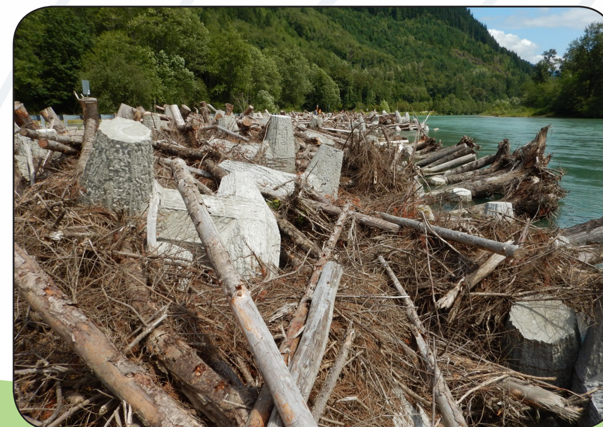
ELJ with dolosse on Skagit River looking upstream 2013.
