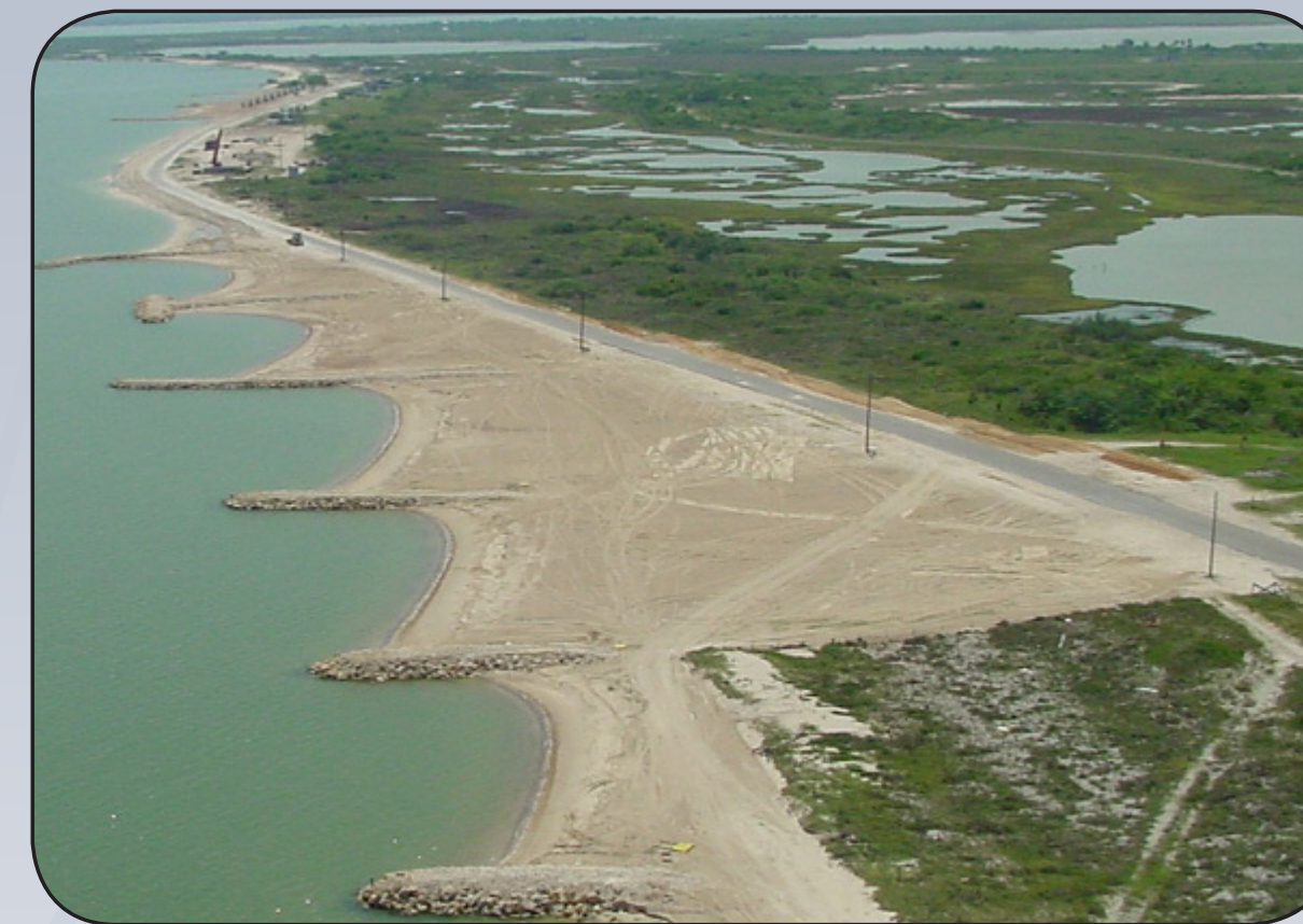
Groins used in a marine setting to control erosion.
