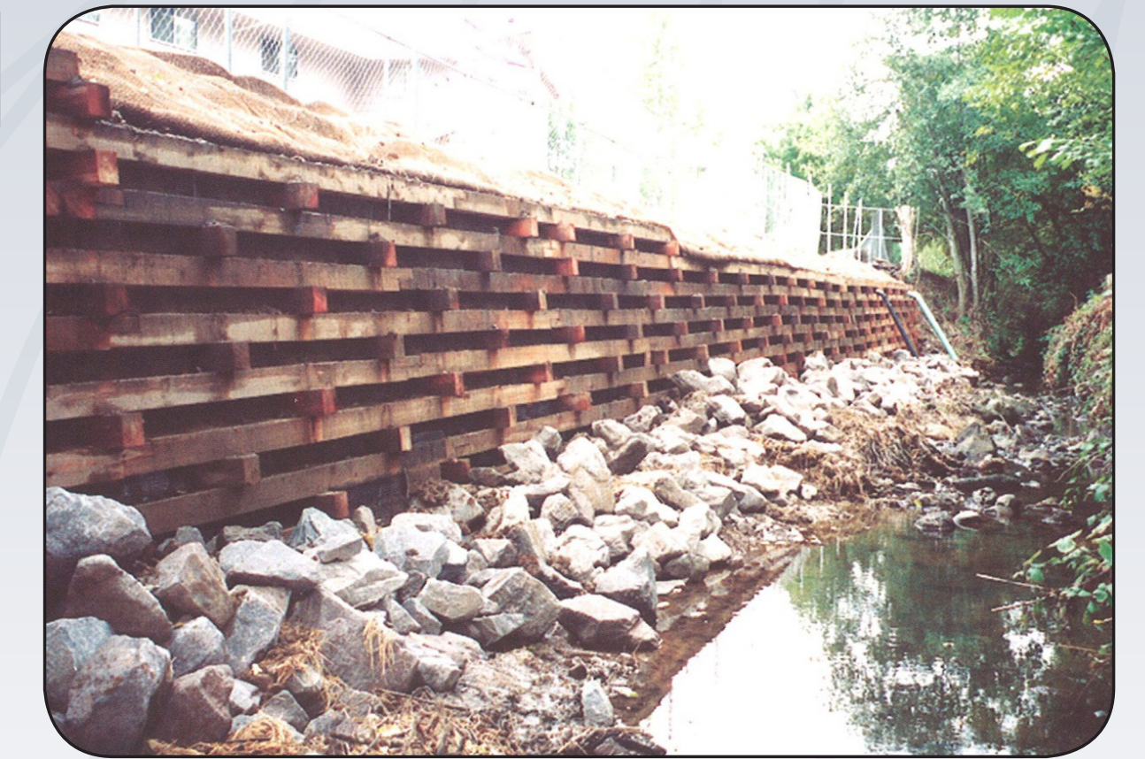
Log crib wall, Fanno Creek, OR.
