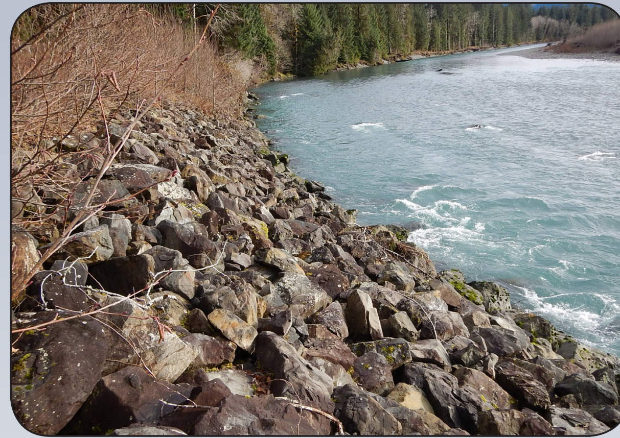
Riprap on the Hoh River, 2014.
