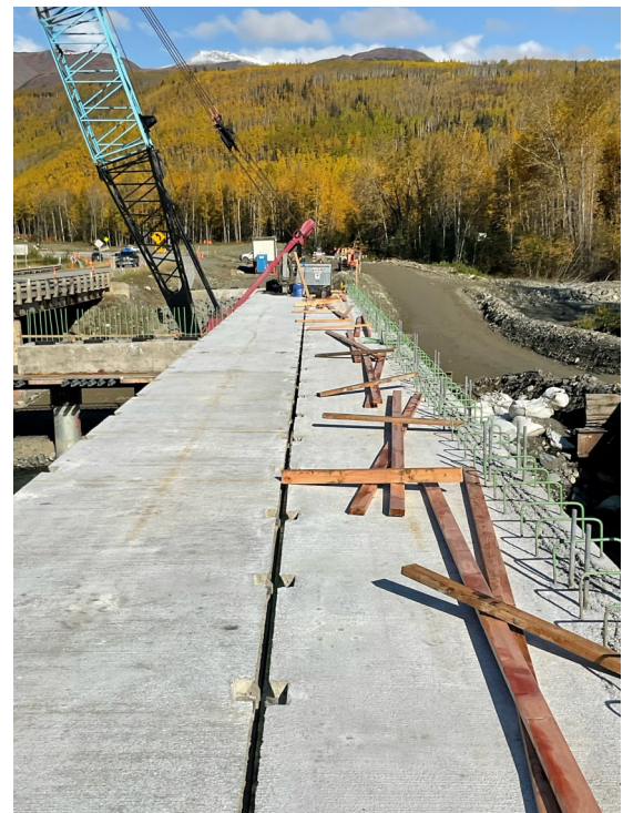
Right: Concrete girders in place on Span 2
