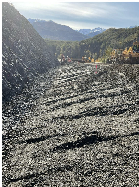
Left: Shaping roadway and ditch slopes
